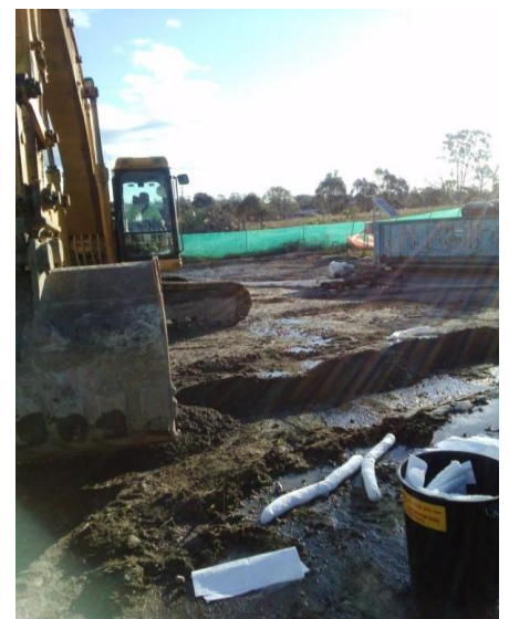
Making a dam with an excavator
